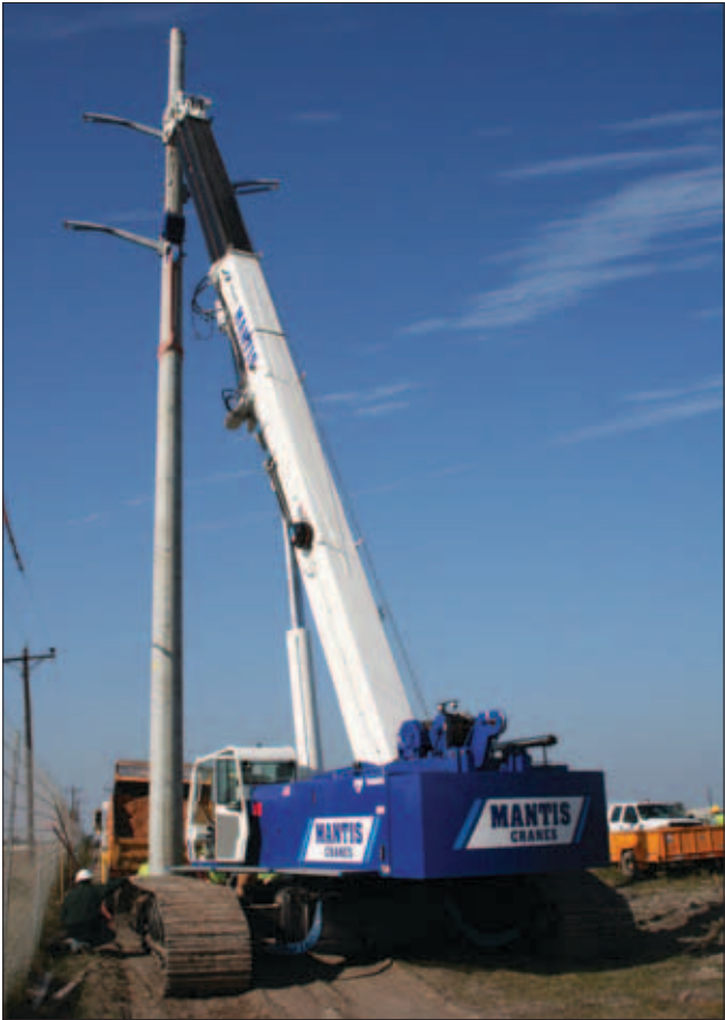
The ability to telescope the boom under full load simplifies the handling and placement of heavy concrete poles.
