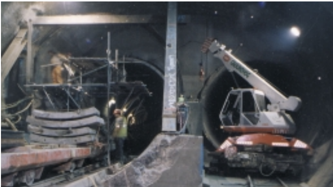
CX-8T – Underground on the Heathrow Express project lifting 1 Tonne tunnel segments into position at a radius of 6.5m with boom at 10m, from adjacent rail position. ▲
