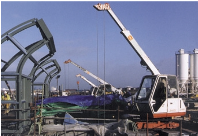
CX-3T ▲ Air-lifted onto sluice gate headings for Shuttering & Formwork duties at Cardiff Barrage
