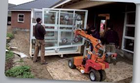
The wide tyres make the lifting device suitable for difficult off-road jobs.
