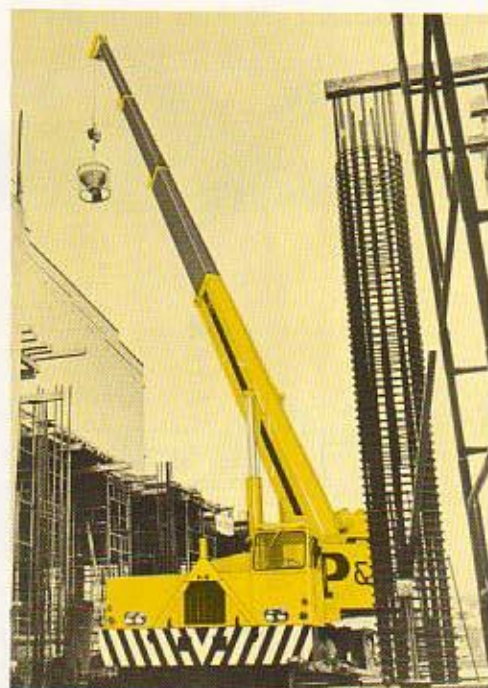
Boom zooms out to full 105' in moments . . . with additional 45' of jib available.
