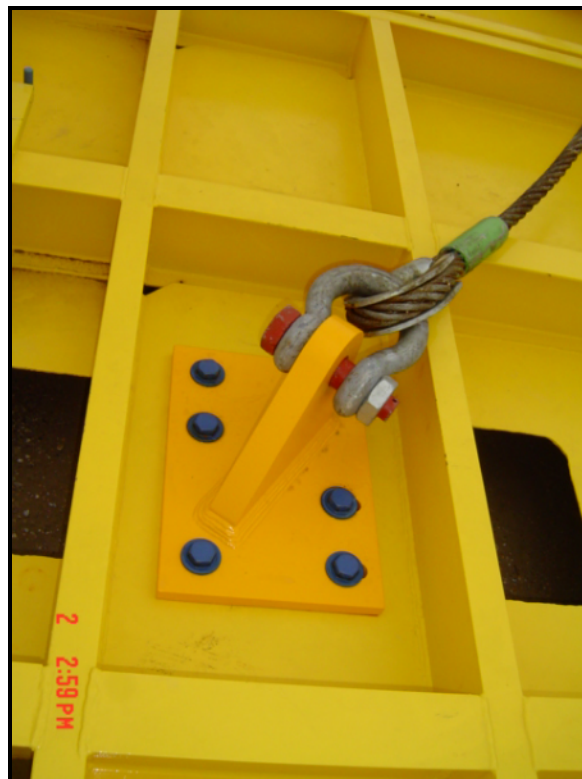
Figure 19 - Lifting Pad Eye and Sling Connection
