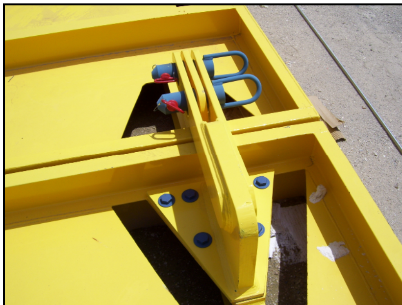
Figure 17 - Bolted and Pinned Hinge Connection
