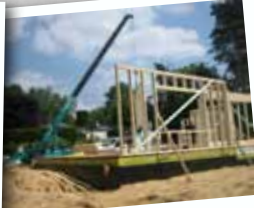
Timber Frame Work
