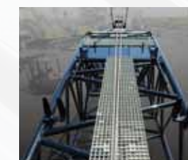
Wider skywalk (made by FRP)
