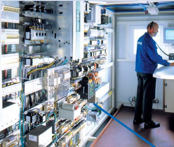
Air-conditioned electrics compartment
