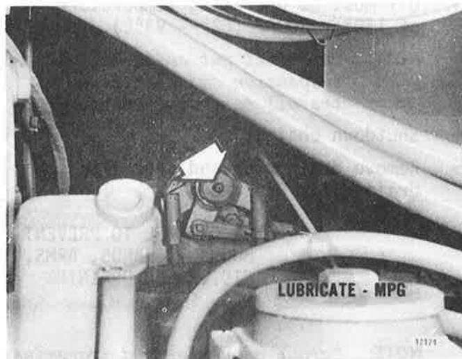
Figure 180 TRANSMISSION SHIFT LINKAGE
