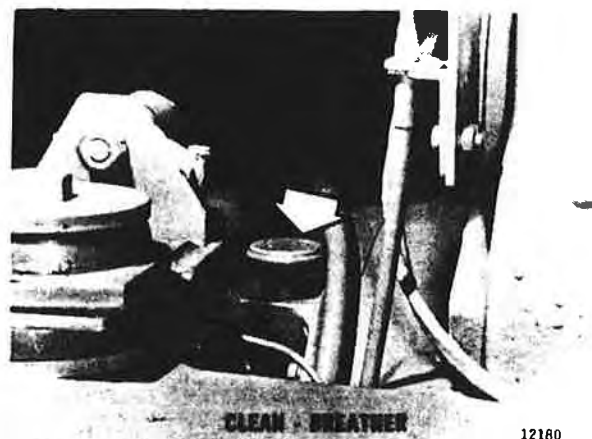
Figure 146 TRANSMISSION AND CONVERTER BREATHES
